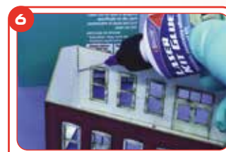
The long reach needle is also ideal for applying the last bit of reinforcing before fitting the roof.
